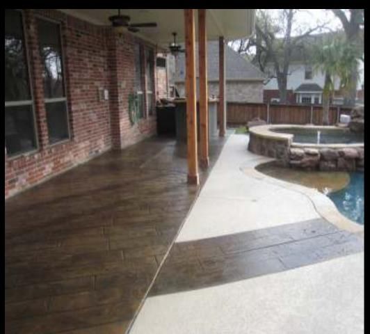
TUSCAN is a textured decorative concrete effect created by applying a thin overlay to an existing or new concrete surface. The Sundek artisan then creates a custom texture on the surface using their trowel and their experience, thus crafting a unique look resembling a deeper stamped concrete overlay.
