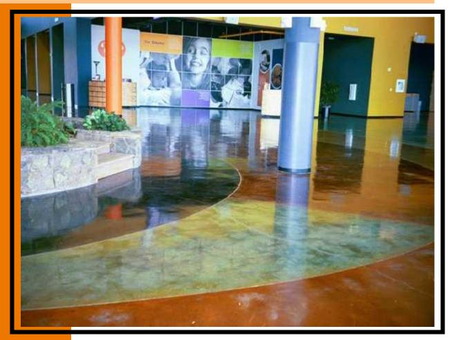
A penetrating, reactive acid based stain for concrete or overlay surfaces.
