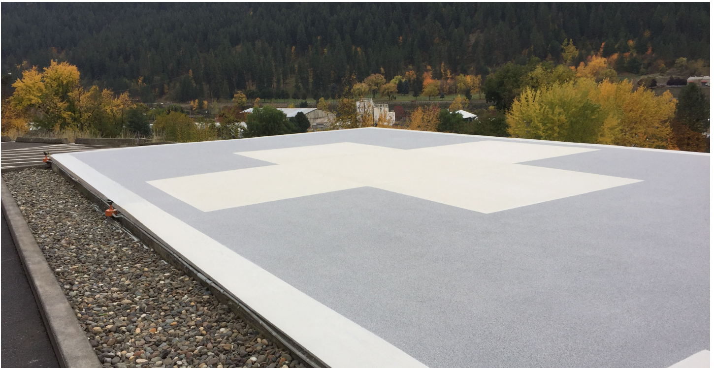
Photograph and installation by Knox Concrete
