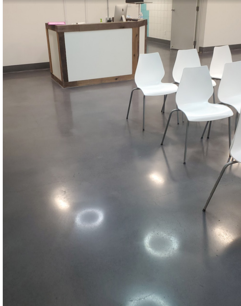
At this youth room in Cross Points Church in Shawnee, KS, Big Red Decorative Concrete installed SunBurn on this surface in addition to hallway surfaces throughout their Religious Educational Building.
